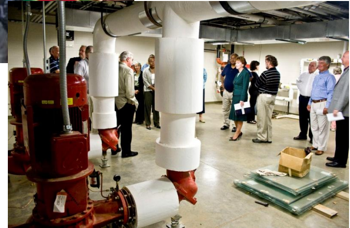
Geothermal HVAC at Mars Hill College
